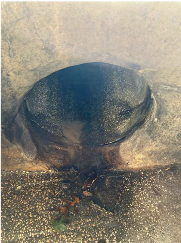
Photo 3 and 4. Crack located at connection of 18" pipe to Structure 11-59. Sediment and groundwater intrusion observed.
