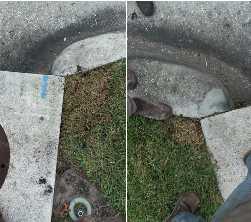
Photo 7 & 8. Completed filling of depression adjacent to inlet.
