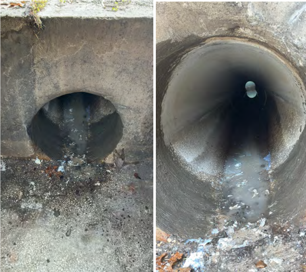
Photo 7 & 8. Completed filling of depression adjacent to inlet.
